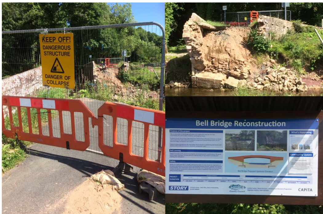
Plate 3: Bell Bridge on the River Caldrew, south of Carlisle, collapsed in late January 2016, as a result of damage sustained during Storm Desmond a month earlier. These images from July 2017 illustrate the closure (stabilisation) of the bridge pending the implementation of the full reconstruction (recovery) project. Note the information board which has been designed to explain the on-going process to the public.
