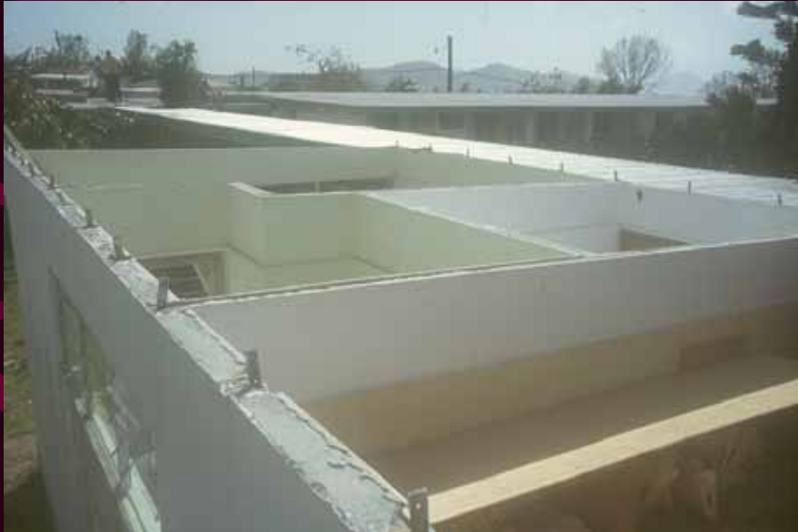
Structure lost in spite of clips
