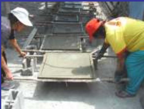
Concrete domes for the roof
