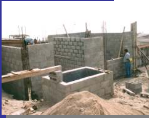
Concrete blocks units in the walls
