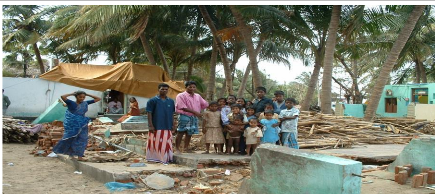
Figure 1: Destruction caused by the tsunami in a village in Nagapattinam district, Tamil Nadu, India (Source: Prathap Tharyan)
