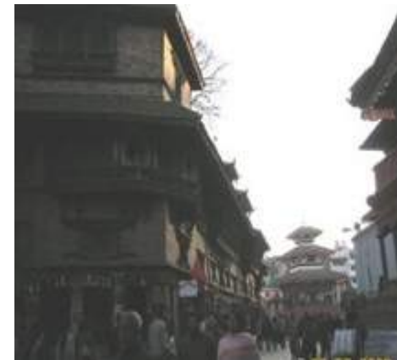
A view of historic city core in Kathmandu which is highly vulnerable to earthquake disasters
