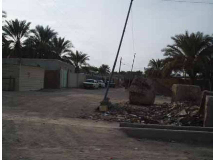
Picture 3. Industrial part of city, across from the steel foundry. Standard bricks and steel shacks. Flat terrain. 10-30 years old.
