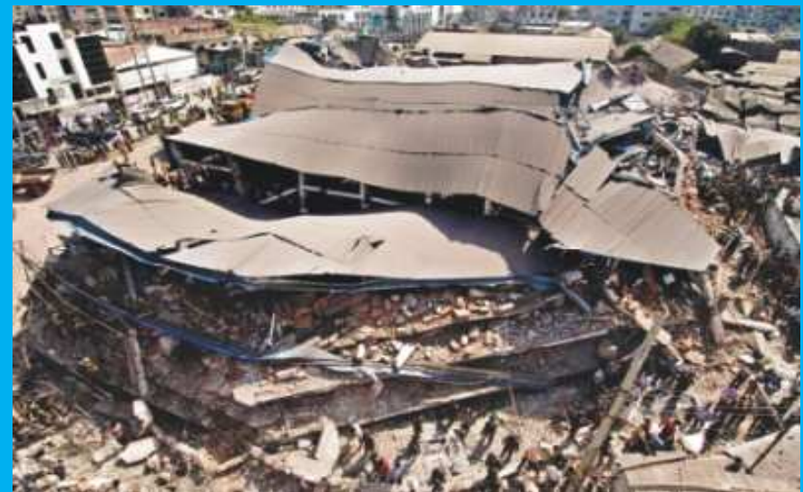
6 story building collapsed- died 21, 25/02/2006
