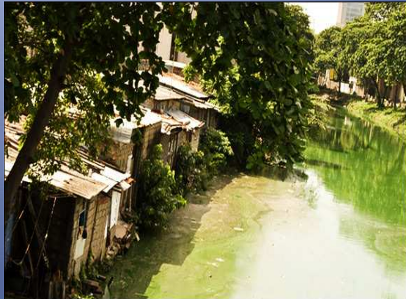
Unauthorised structures on a canal reservation
