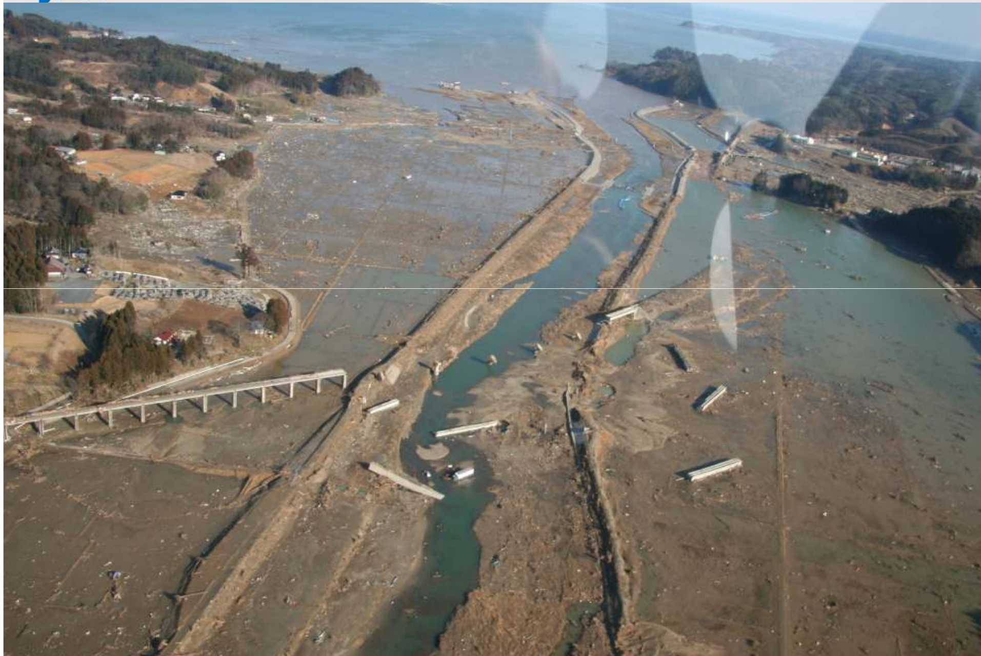
Railway Bridge washed away by Tsunami wave at Tsuyagawa Bridge, Kesennuma Line (Photo: JR East)
