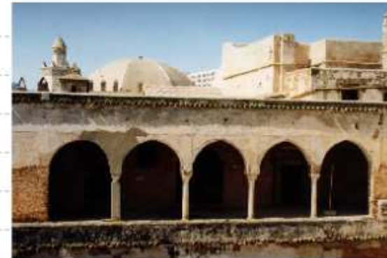
The Horseshoe-pointed arches (Arcads).
