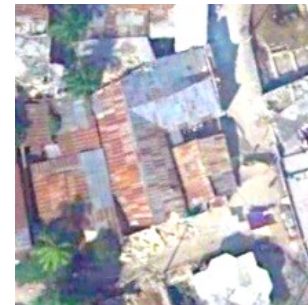
GRADE 4: Very heavy damage
