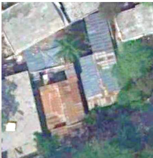
GRADE 3: Substantial to heavy damage
