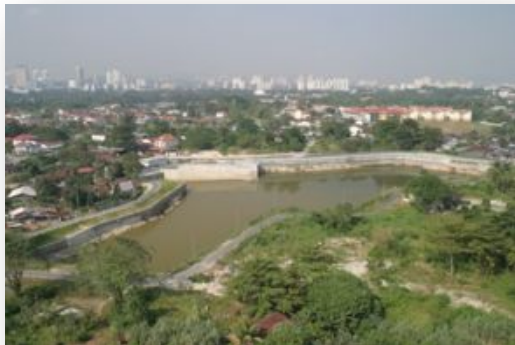
Flood detention pond with pumping facilities
