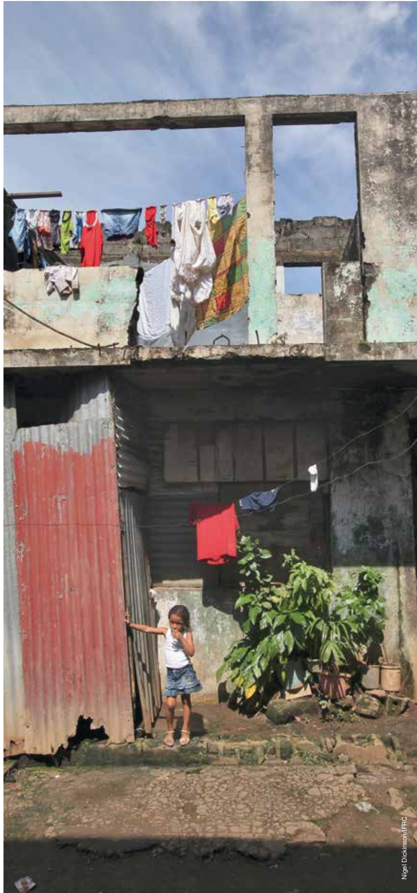
Families in the Boer district, Managua, Nicaragua, squat in unsafe buildings destroyed by the 1972 earthquake.
