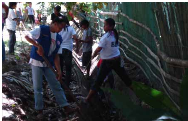
Disaster mitigation: cleaning drainage canals, Palawan, Philip.2009
