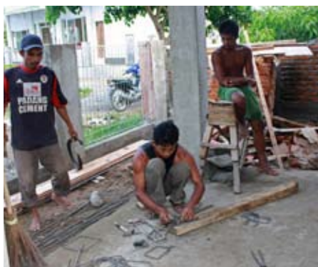
Homeowners learn from construction wokers
