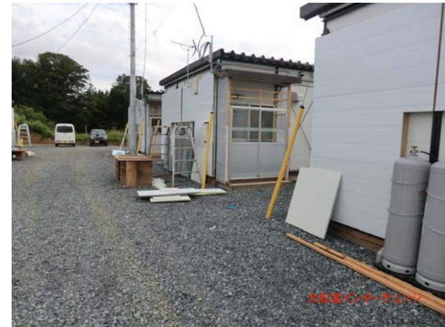
Additional work to attach heat insulation panel.
