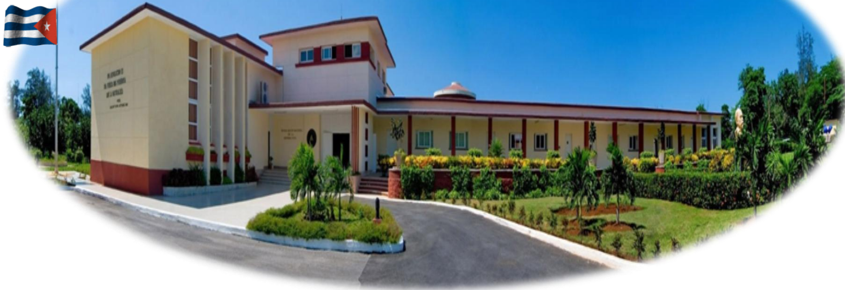
Cuban Civil Defense Headquarters (CD-HQ)
