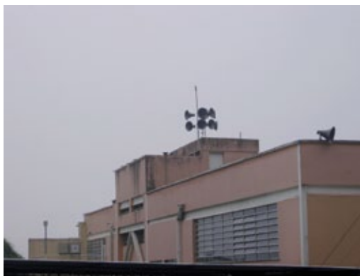
Photo 4.9: Sirens and rain meter in the remote alarm unit in the Morro da Formiga community. The equipment was installed on the terrace of a local school, also used as a temporary refuge in the event of extreme weather.
