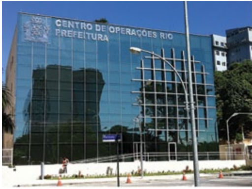
Photo 4.11: CO-RIO, City Government Operations Center
