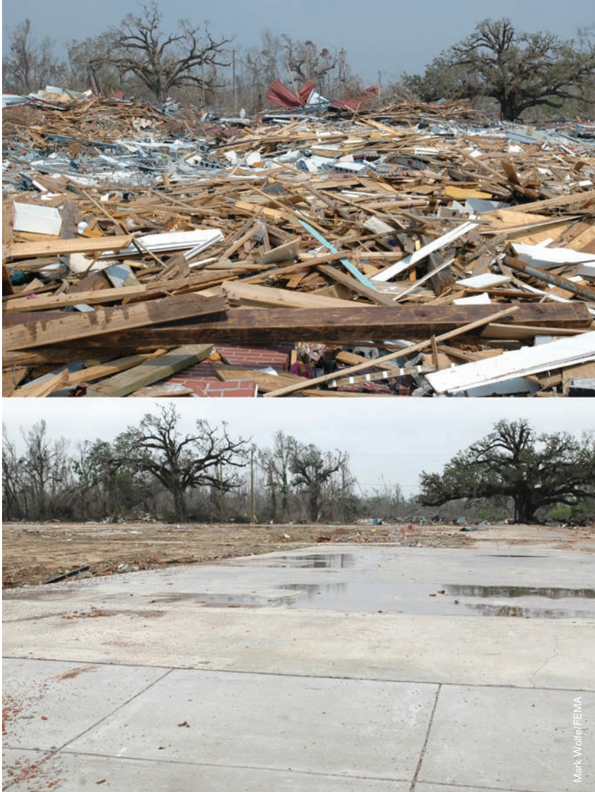
The debris from Pass Christian Middle School in Mississippi before (above) and after cleanup. The school was destroyed by Hurricane Katrina in 2005.
