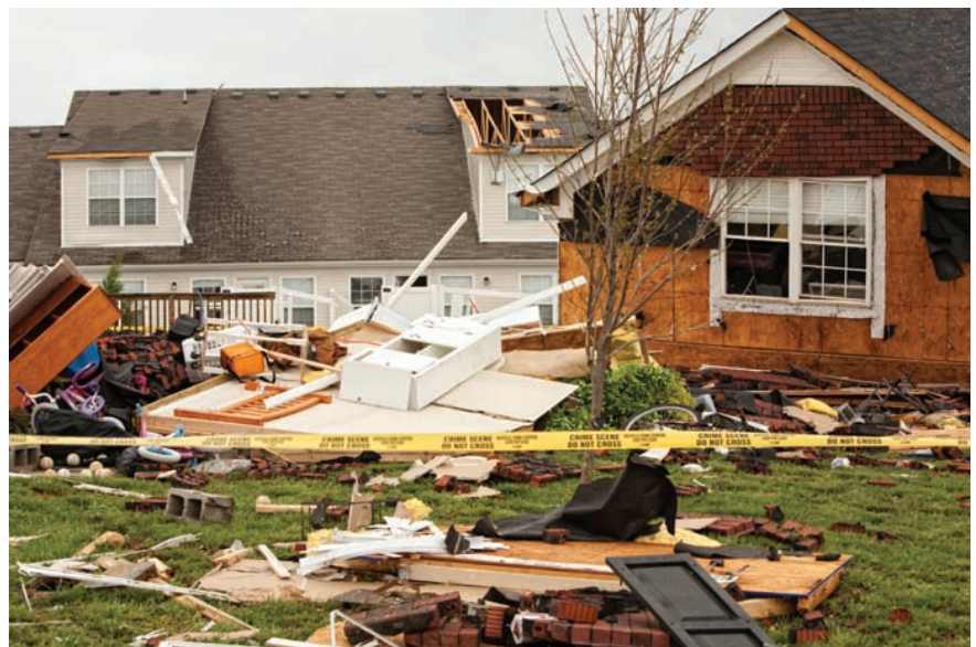
The town of Murfreesboro, Tennessee, suffered severe damage from a tornado in April 10, 2009.
