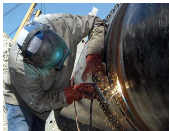
Construction of the BTC pipeline in 2004
