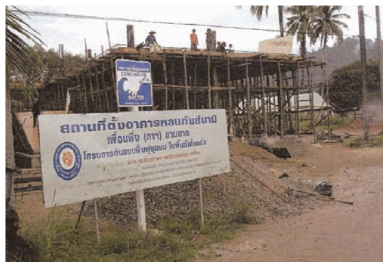
Evacuation Building Place
