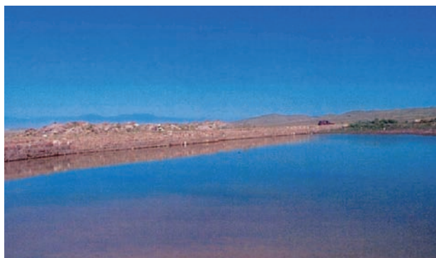
Fig. 2 The view of the Eghnik dam from upstream
