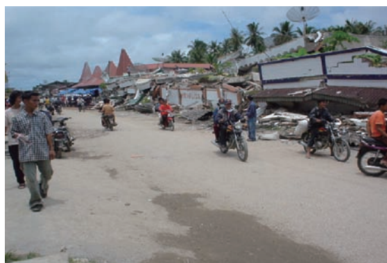
Destructive earthquake in Nias on March 28, 2005.
