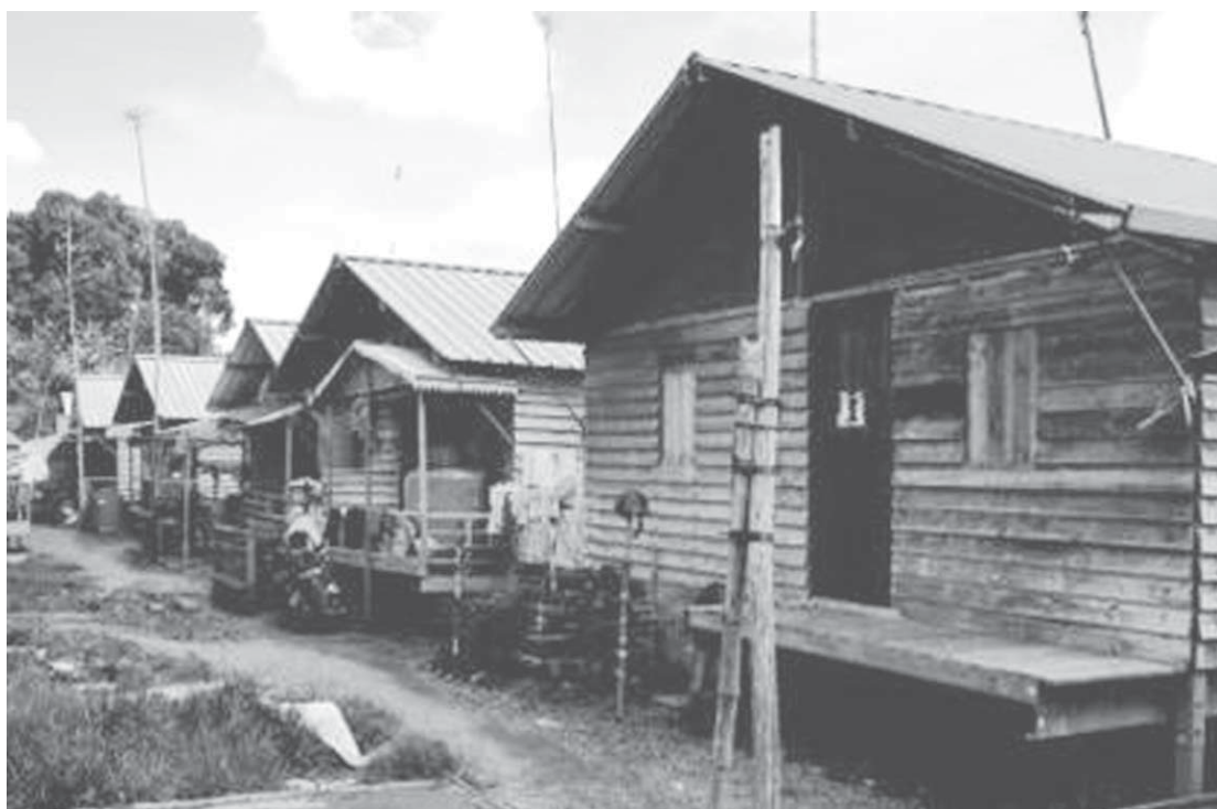
Figure 4: Simple houses built for tsunami survivors at Terbih village in the vicinity of Jantho, the capital of Aceh Besar District. Another 25 participants of the first UNESCAP training workshop came from this refugee camp.
