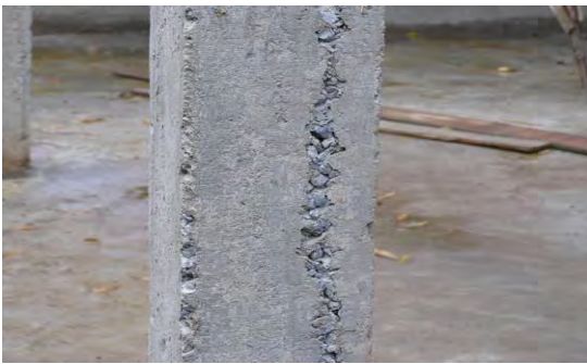
Figure 5: "Honeycombing" - caused by shoddy, cost-cutting construction practices
