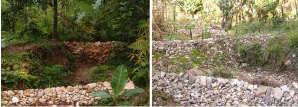
Gully plugs in the ravines
