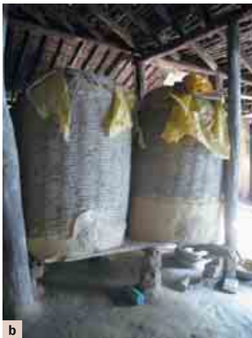
Figure 13: Different types of grain store: a) Outside grain store with a brick base, Phoolparasi VDC, Sarlahi District; b) grain store made of bamboo inside a house, Singyahi VDC, Mohattari District; c) grain store made of mud and poles inside a house, Singyahi VDC, Mohattari District
