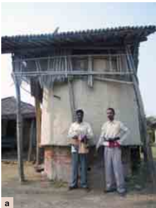
Figure 13: Different types of grain store: a) Outside grain store with a brick base, Phoolparasi VDC, Sarlahi District; b) grain store made of bamboo inside a house, Singyahi VDC, Mohattari District; c) grain store made of mud and poles inside a house, Singyahi VDC, Mohattari District
