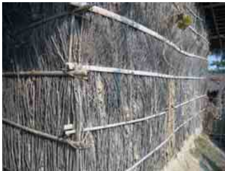
Figure 6: Walls of a local house made out of dried pulse plants, Kaitarait VDC, Dhunusha District
