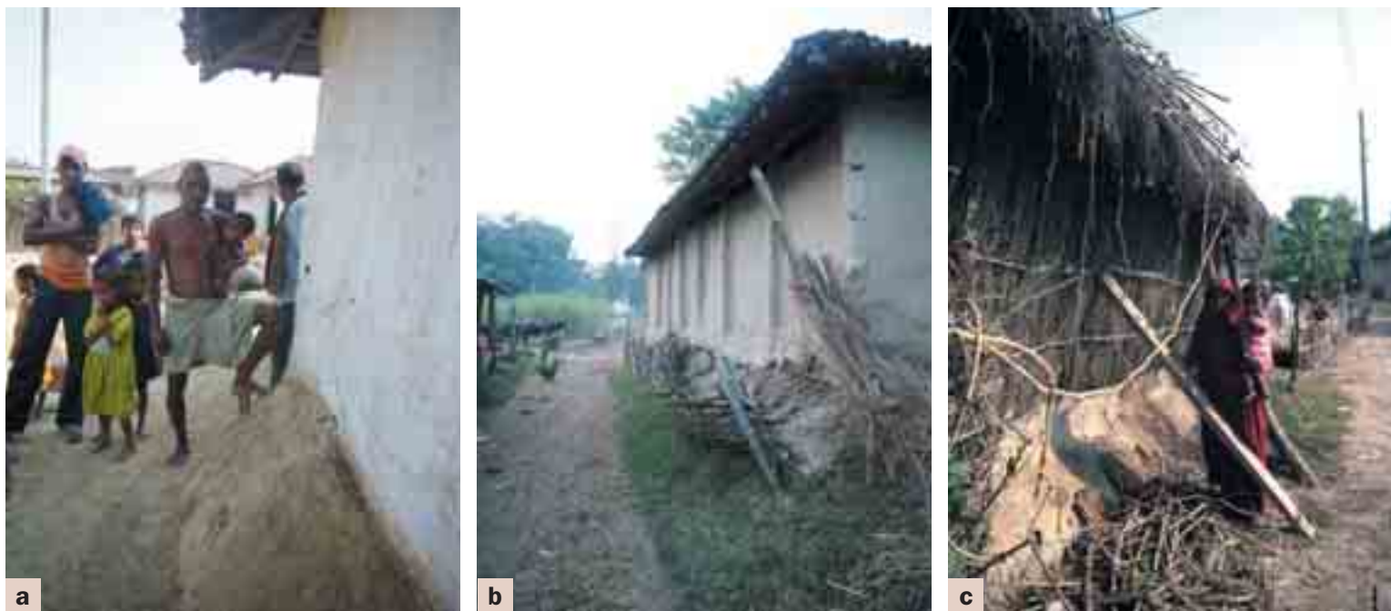
Figure 9: Strengthening and protecting walls and wall foundations: a) foundations protected with piled up mud, Katarait VDC, Dhanusha District; b) foundations protected with a bamboo fence and mud, Katarait VDC, Dhanusha District; c) wall made of bamboo, mud, and dried pulse plants supported by a wooden beam, Seurai VDC, Dhanusha District
