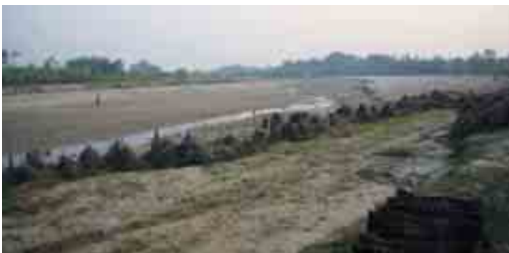
Figure 19: Embankment made out of bamboo constructed by a local NGO using local knowledge and local material. Phoolparasi VDC, Sarlahi District
