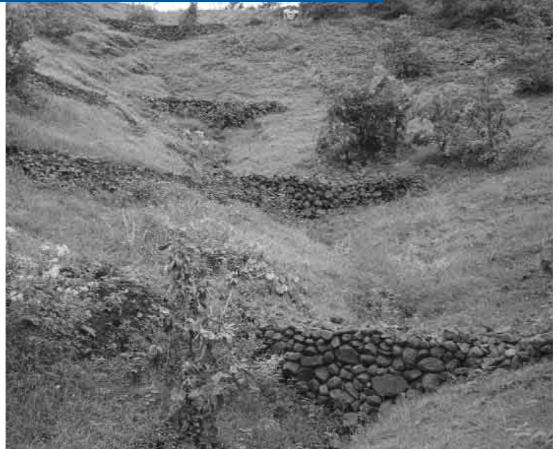
Gully plugs, Nagzari, India (October 1999). Photo courtesy of WOTR
