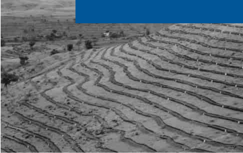
Continuous contour trenches, Chincholi, India (December 1998). Photo courtesy of WOTR
