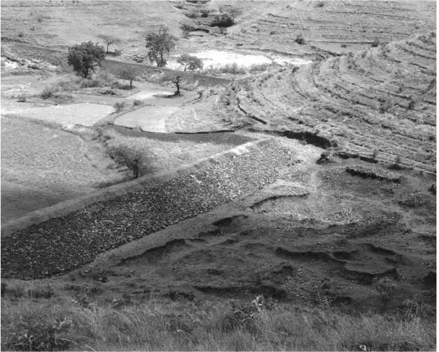
Nala Bund, Chincholi village, India (October 1997). Photo courtesy of WOTR
