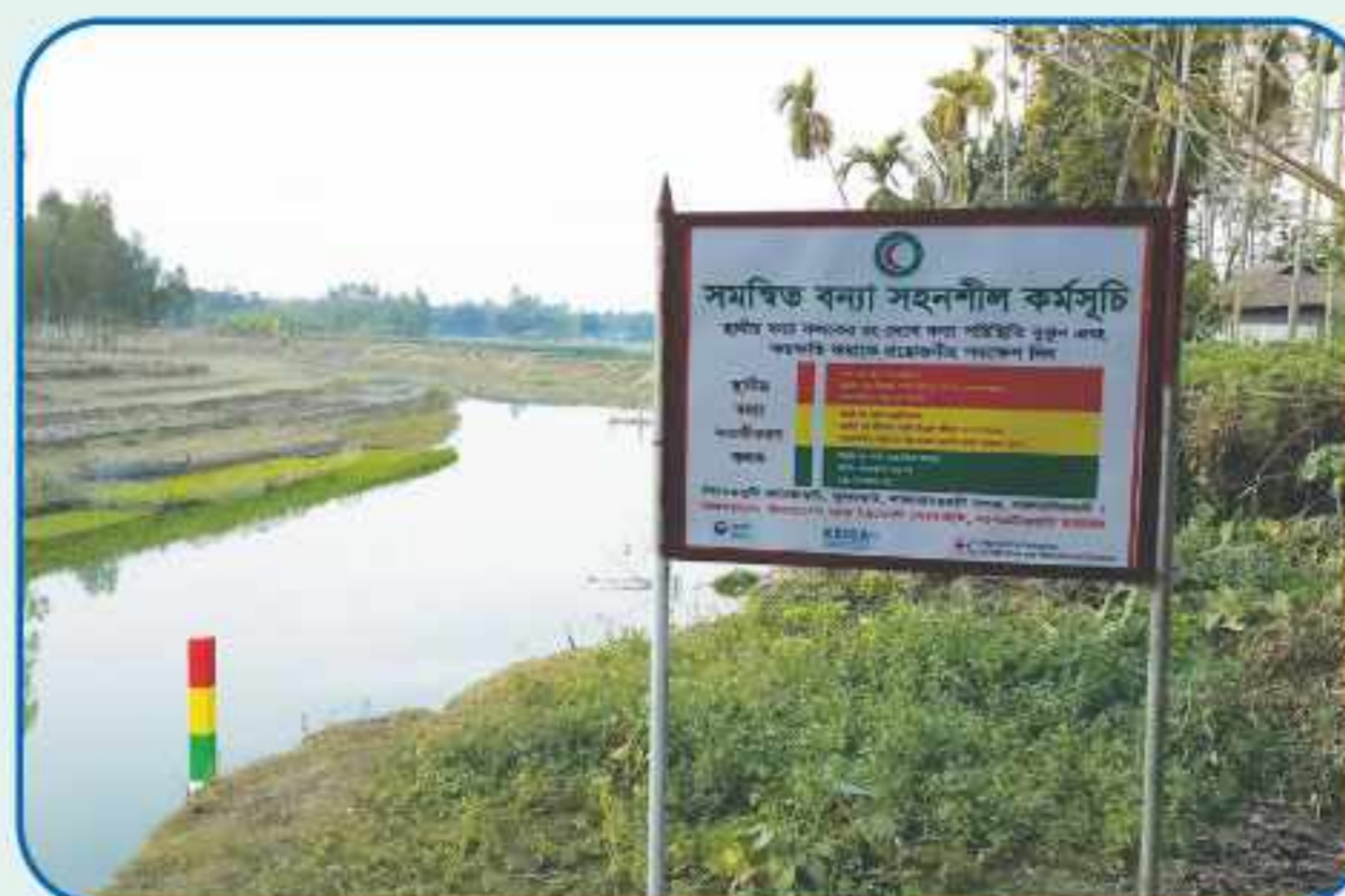
Flood marker with explanatory signboard, at Shiber Kuti community beside the Ratnay river, Lalmonirhat (Photo: BDRCS)
