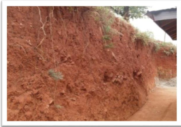
Figure 4: Digging of foundations on steep slopes with thick soils.
