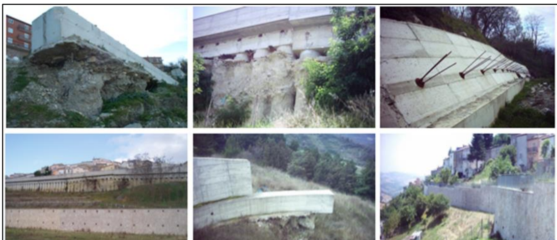
FIGURE 6. Examples of ineffective stabilisation measures realised on the unstable slopes.
