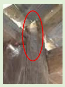
Note: 3 mmm thick metal strap, Minimum four numbers of 50 mm long nails (Fe250) with Floor member and Minimum four numbers of M16 grade expansion bolts with walling material
