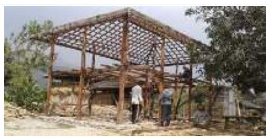
Figure is shown in traditional of timber framed structures in Siwalik range.
