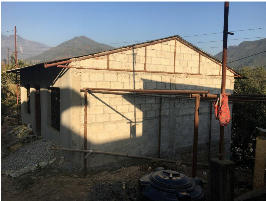
HCB house with steel truss for roof in Nuwakot.
