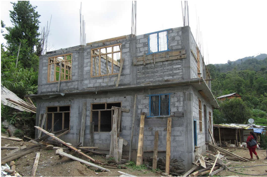
RC frame building with HCB infill in Dolakha.
