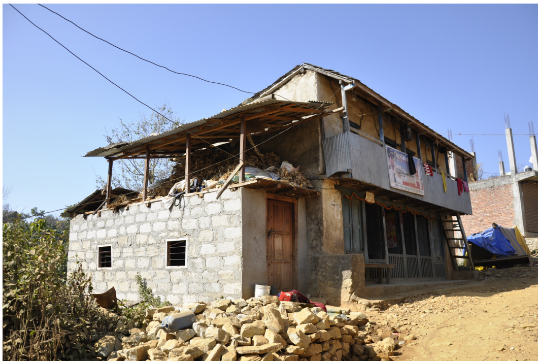
HCB extension to a stone masonry house in Dhading.
