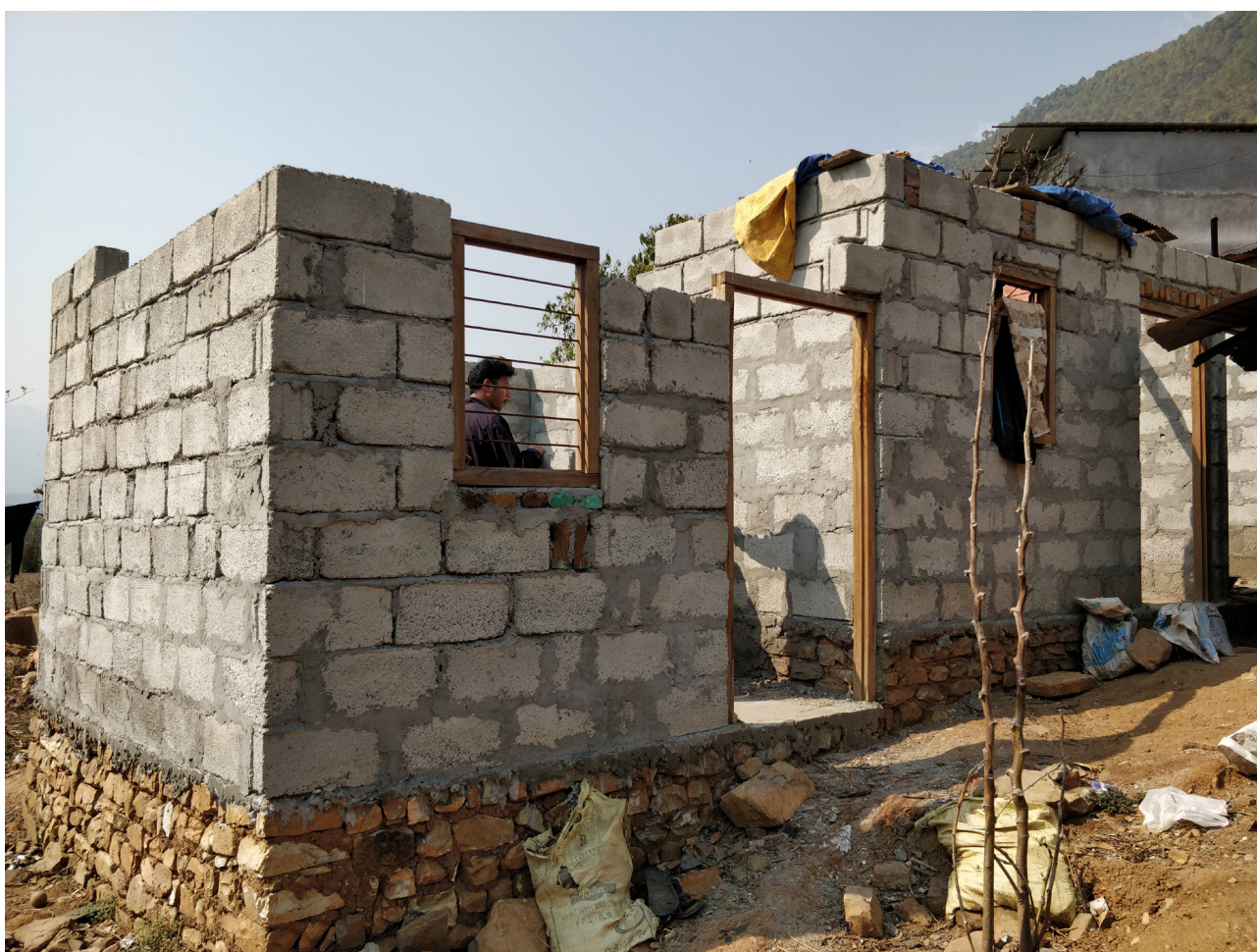
Lekhnath Municipality, Pokhara, Kaski: one of more than 600 houses that have been constructed using hollow concrete blocks in this area. Households in the area regularly ask the GoN engineers for designs for HCB houses. The engineers have been providing the designs from the DUDBC Design Catalogue Volume 2, but households are not building according to these designs.
