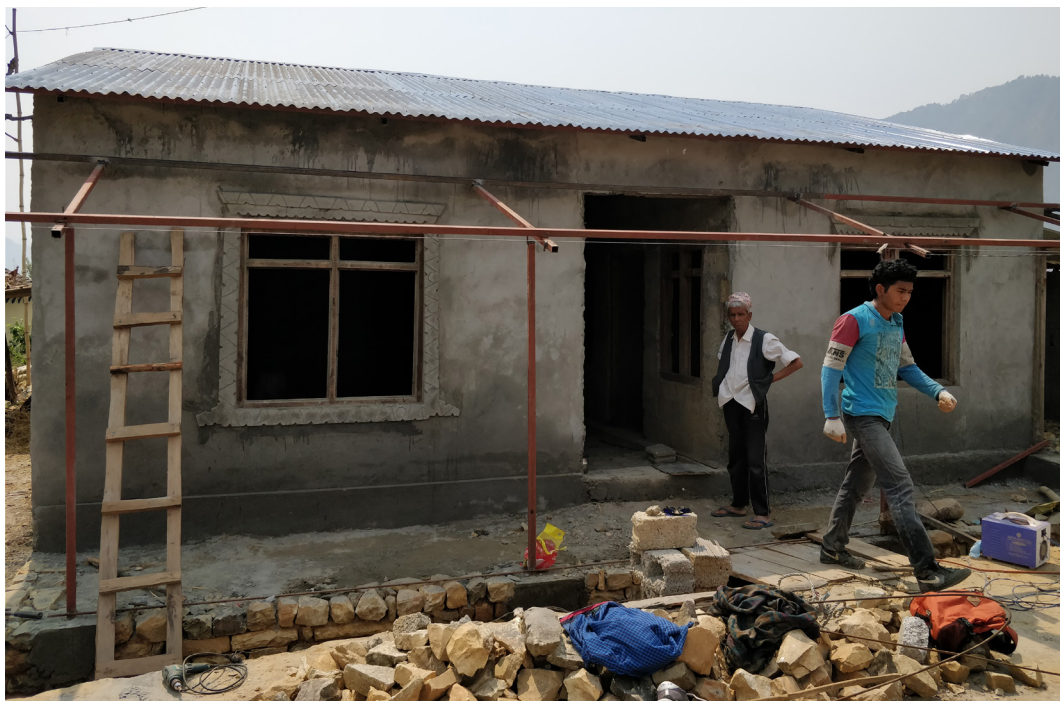
Modi Rural Municipality, Ward No. 6, Parbat (one of the 18 moderately affected districts): Purna Bahadur BK started construction of his 5 room house, with steel frame structure and hollow concrete blocks for the infill walls, just 1 month after the 2015 earthquake. He is still going through the grievance mechanism and he didn't know that this house would not be in line with government standards as there no guidance available previously and the inspection engineers have just been deployed.
