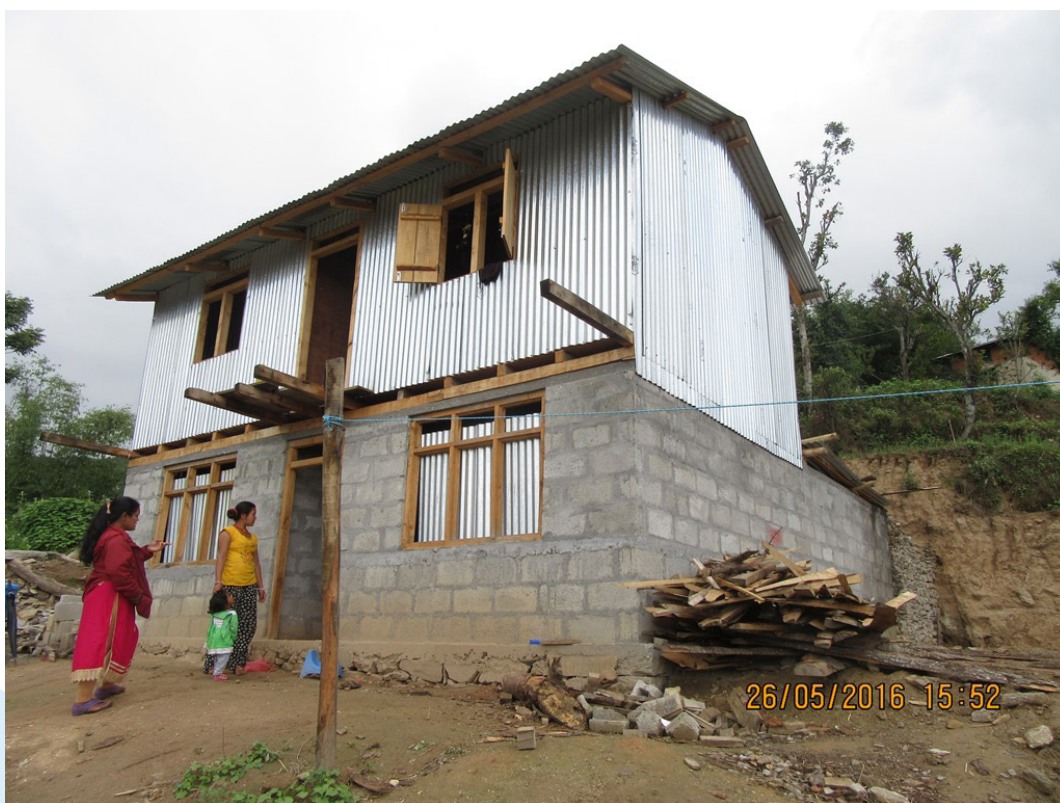
Hybrid construction in Dolakha with HCB construction on ground floor and timber and CGI first floor.
