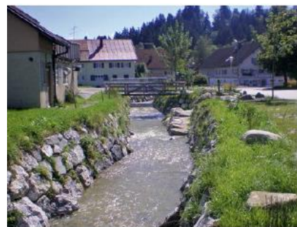
Longitudinal protection measures: Concrete wall (left), stone wall (right) (Rimböck, Höhne, Mayer, & Wolter-Krautblatter, 2015)
