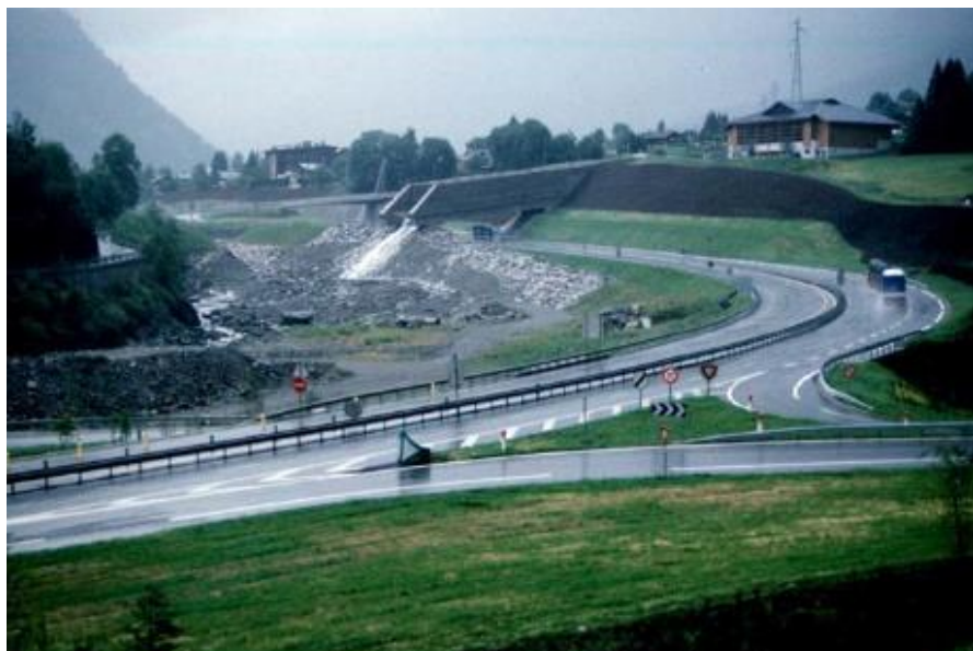
A debris flow bridge, protecting a road in France (Unknown, ?)
