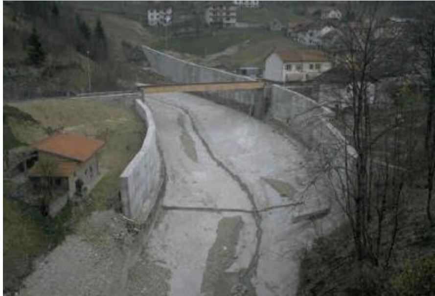
Shooting channel conduction mud flows through a village in Italy. By diverting water into it, the shooting channel can be flushed after events (Unknown, ?)
