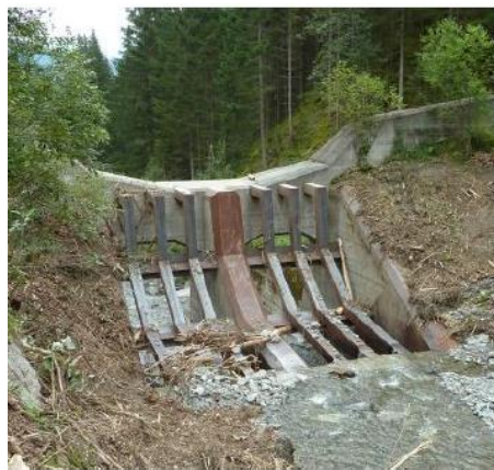
Large slot grill barrier (Mazzorana, et al., 2015)
