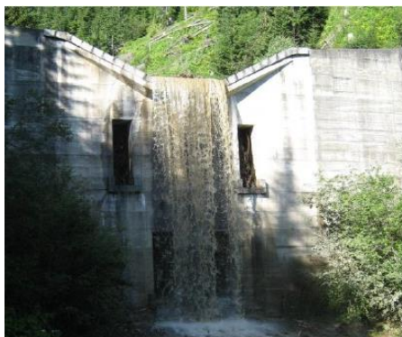
Large silt trap barrier (Mazzorana, et al., 2015)
