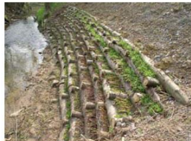
Engineer-biological method (tree wall) (Jany & Geitz, 2013)
