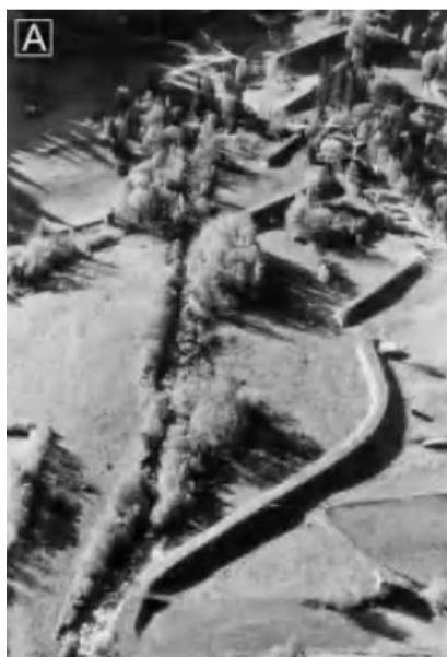
Left: Several conduction dykes in a torrent fan (Bergmeister, Suda, Hübl, & Rudolf-Miklau, 2009)
