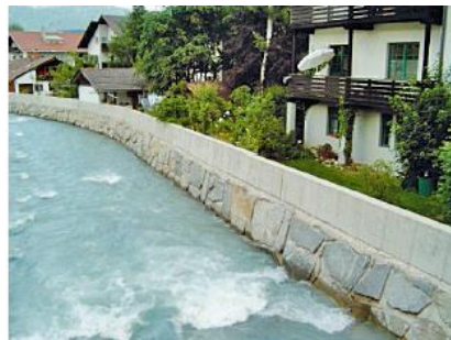
Longitudinal protection measures: Concrete wall (left), stone wall (right) (Rimböck, Höhne, Mayer, & Wolter-Krautblatter, 2015)
