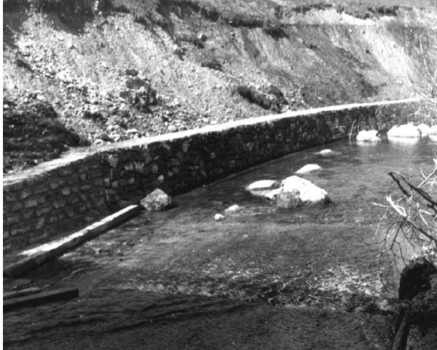
Longitudinal toe slope stabilization (Jakob & Hungr, 2005)
