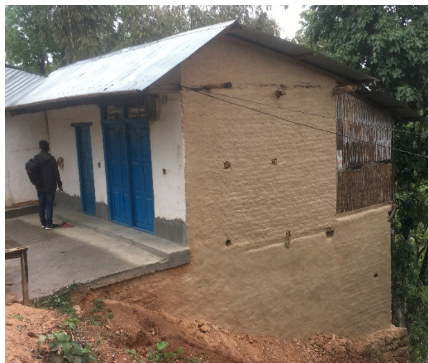
Khandbari Municipality ward-8, Sankhuwasabha: non-compliant house constructed with stone and mud mortar masonry on the ground floor and sun-dried bricks for the first floor. This house was constructed before technical assistance in the district. The home owner has received the first tranche and applied for the second.
