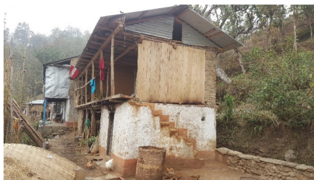
Diktel Rupakot Majhuwagadhi Municipality ward-I, Khotang: non-compliant hybrid structure with ground floor having stone and mud mortar masonry walls on three sides with one open side and the first floor walls are constructed with timber and CGI sheets. The home owner built the house in early 2017 with no technical support. They have applied for the second tranche of the reconstruction grant but will not be able to receive it without carrying out corrections.
