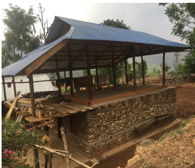
Chainpur Municipality ward-II, Sankhuwasabha: non-compliant Hybrid Structure with ground floor built in stone in mud mortar masonry and first floor with timber frame and open walls for now. The house was completed in early 2017 with no technical assistance. The home owner has received just the first tranche of the housing reconstruction grant.
