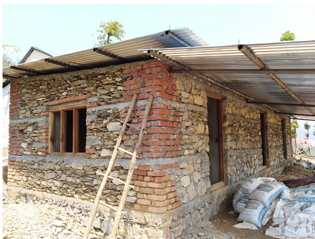
Santoki Kumar, Sandhikhark 7, Markakhola, Arghakhanchi: hybrid structure with stone and brick masonry and a mix of mud and cement mortar. The owner brick masonry in the corners to reduce labour requirements and constructed the rest of the house himself. The wall to roof connection is poor and the DLPIU engineer listed the house as non-compliant. However, the engineers are not able to support with implementing correction and exception techniques as they have not received any training on this.
