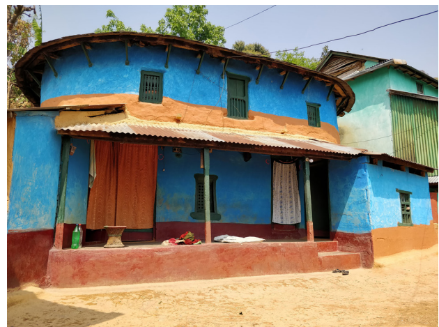
Waling Municipality (ward-5), Syangja: the home owner reduced their circular 3 storey house to one and a half storeys after it was damaged by the 2015 Gorkha earthquake. They are now planning to construct a new house and the government technical staff have said that the damaged house will have to be demolished before the third tranche of the GoN housing reconstruction grant can be released.
