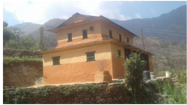
Jayamuni Municipality (Ward-9), Baglung: non-compliant stone and mud mortar masonry house constructed without technical guidance. The household have received the first tranche of the GoN housing reconstruction grant but they now need to apply corrections based on the Corrections and Exceptions Manual to receive the remaining tranches.
