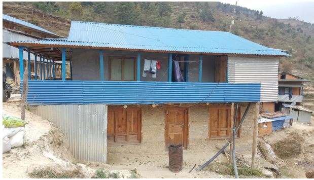
Solu Dudhkunda Municipality ward-11, Tignasa Solukhumbu: non-compliant Hybrid Structure built in early 2016 with no technical assistance. The ground floor is stone and mud mortar masonry and the first floor is timber frame with CGI sheets. RCC bands have been used at the plinth and timber bands at the lintel and sill level and the openings are not appropriate. The home owner has just received the first tranche of the housing reconstruction grant.
