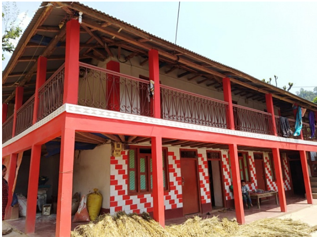
Arghakhanchi: hybrid structure using multiple materials.
