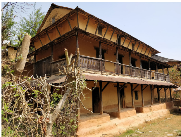
Waling Municipality (ward-5), Syangja: this stone and mud mortar masonry house has survived three earthquakes; one in 1990 B.S., one in 2045 B.S., and one in 2072 B.S. The house is still standing despite the earthquakes and being more than 80 years old. The construction quality is quite good with support from timber bands at floor and roof level i.e. 2 bandings per floor.
