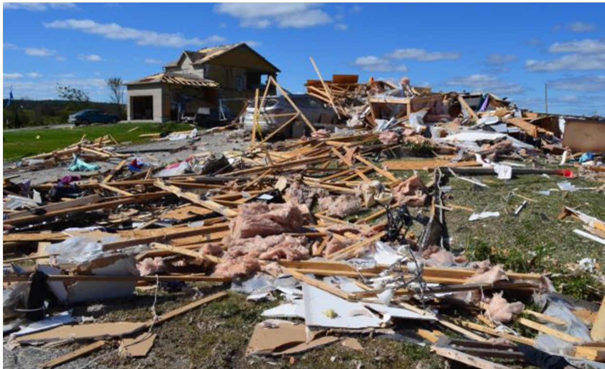
Figure 6. EF3-rated tornado damage in Dunrobin, Ontario. The tornado that caused this damage was the strongest of the six tornadoes that day.
