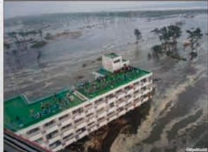
Arahama Elementary School Flooded by the Tsunami
