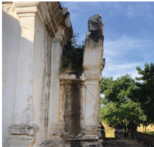
Figures 6 and 7. Slope Stabilization Measures Completed by MOTC (Approximately 2005) and Rotation of the Façade at Thet Kya Muni, Bagan (December 2017)
