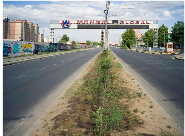
Photo 4: Paved Road, Ulaanbaatar, Mongolia
