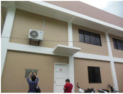
Building provided to the women associations supported by JICA (Photo: July 2015)
