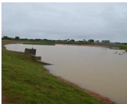
Reservoir built in Vilaveduwani GN with Oxfam assistance (Photo by Oxfam)
