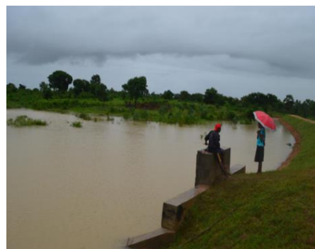
Reservoir built in Vilaveduwani GN with Oxfam assistance (Photo by Oxfam)
