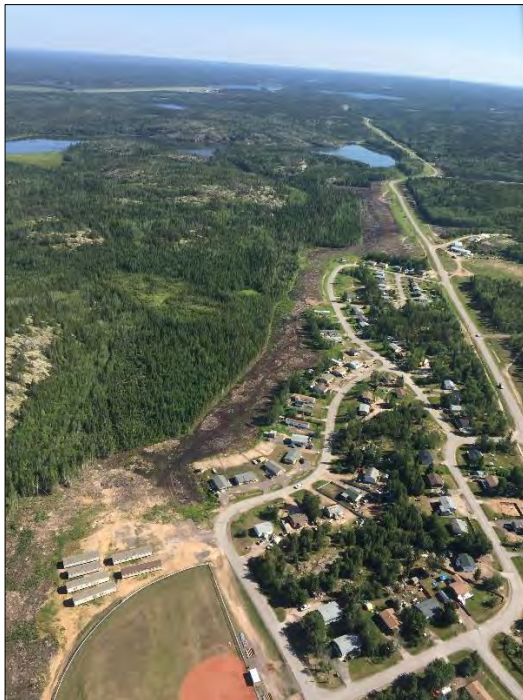
Completed Vegetation Management Areas FB7 & FB8
