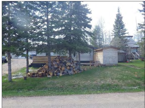
Inadequate Priority Zone 1 from Combustible Piles/Outbuildings
