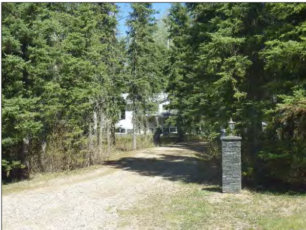
Inadequate Priority Zone 1 Clearance from Forest Fuels
