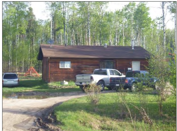
Inadequate Priority Zone Clearance from Surface Fuels
