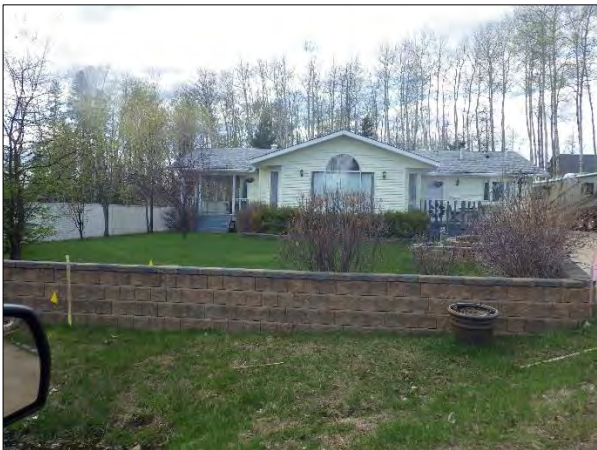
Inadequate Priority Zone 1 from Ornamental Fuels
