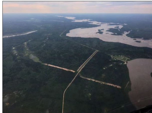
Completed Vegetation Management Areas FB1, 6, 14, & 15
