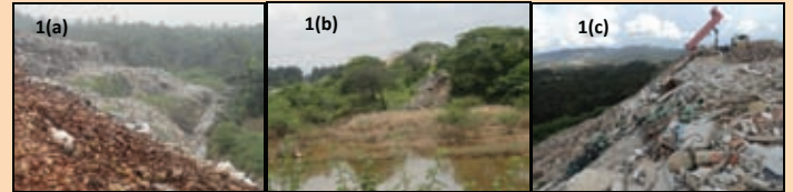
Figure 1. Examples of landfill sites in Selangor that are located on three different settings including (a) coastal, (b) floodplain and (c) on hill slope.
