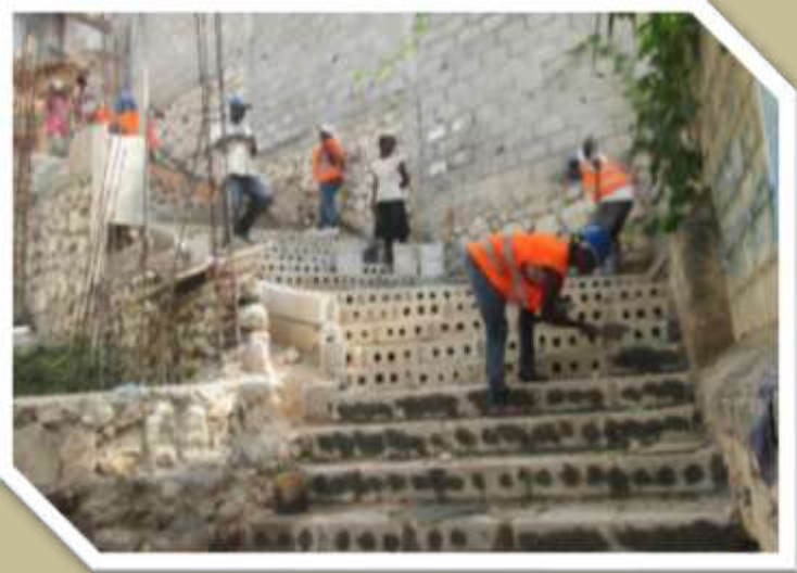
Example of small scale mitigation works, Credit: Goal, 2016
