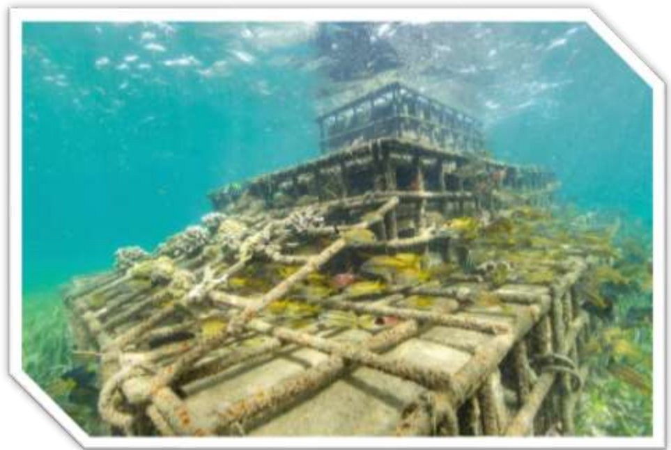
Installed hybrid reef (man-made structure with coral transplants), Credit: TNC, 2016
