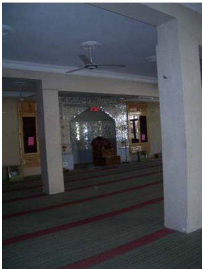
Mosque (note reinforcing pillars)
