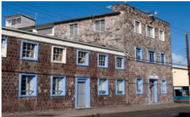
24hr Tsunami Monitoring Police Headquarters, Basseterre
