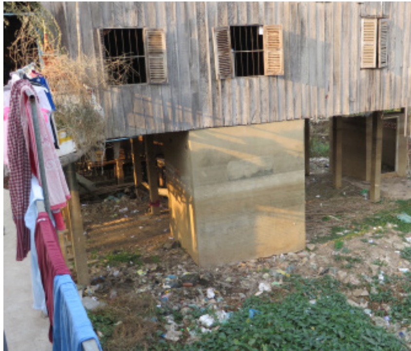
Figure 19: Earth/mud foundations in Chamrouen. Sediments on structure mark flood-water levels
