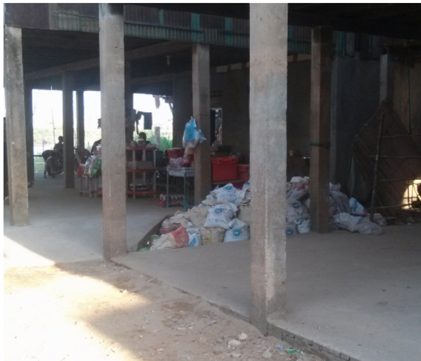
Figure 20: Strengthening of houses with concrete foundations and building materials in Borei Doemsrol
