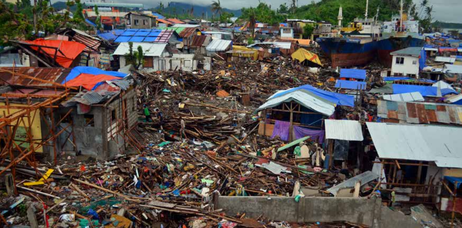
Typhoon Haiyan Damage, Tacloban. Photo credit: Tigeryan
