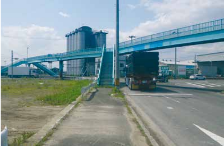
Figure 8a. Pedestrian bridge in Natori. (Suppasri, 30 May 2012)
