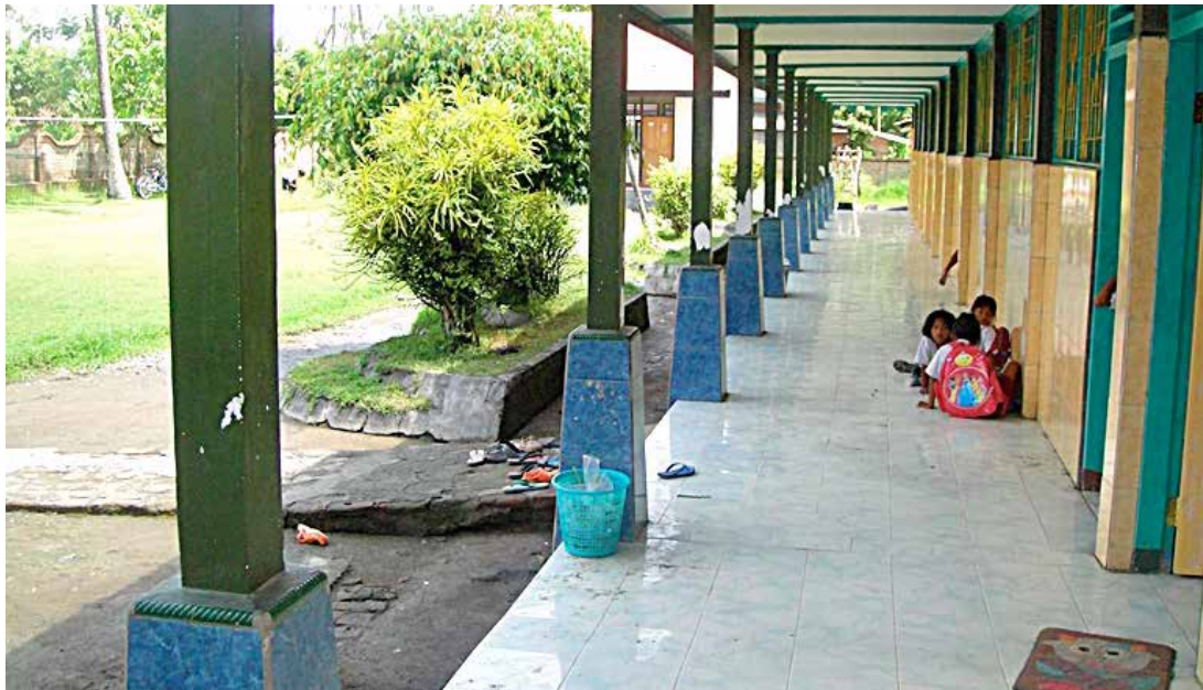
The terrace coloumn of elementary school (SD) 7 Kuripan reinforced with steel bars.
