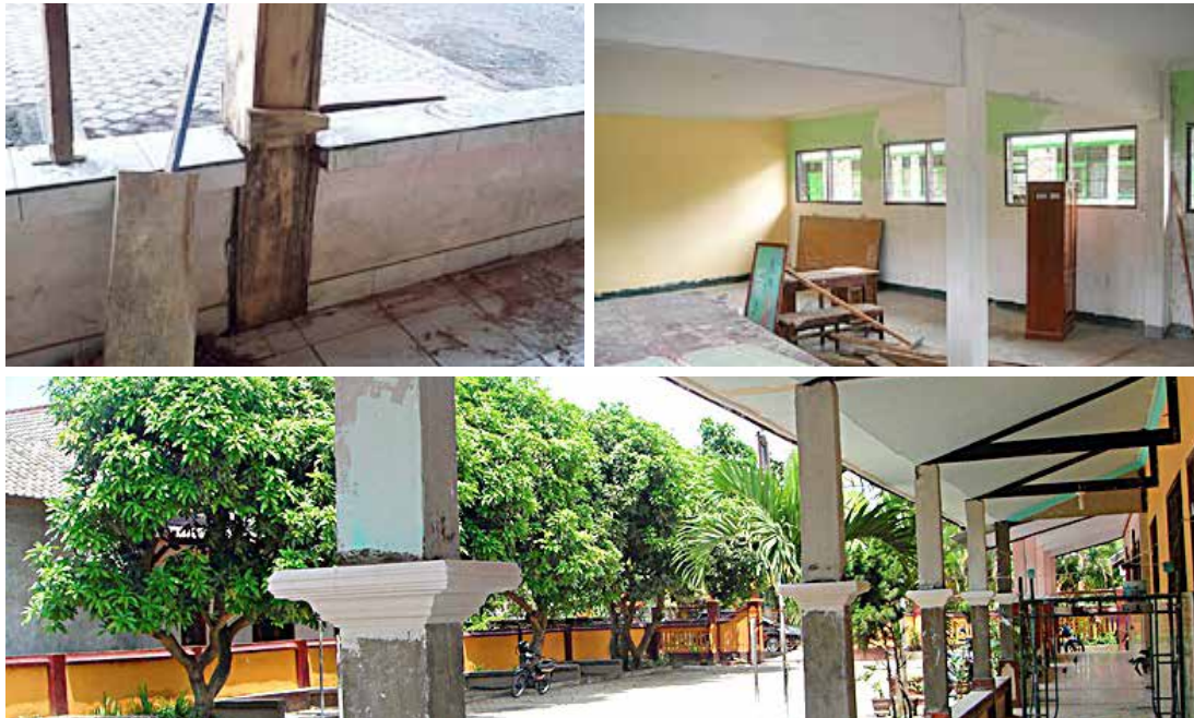
Reinforcement of school building structure.
