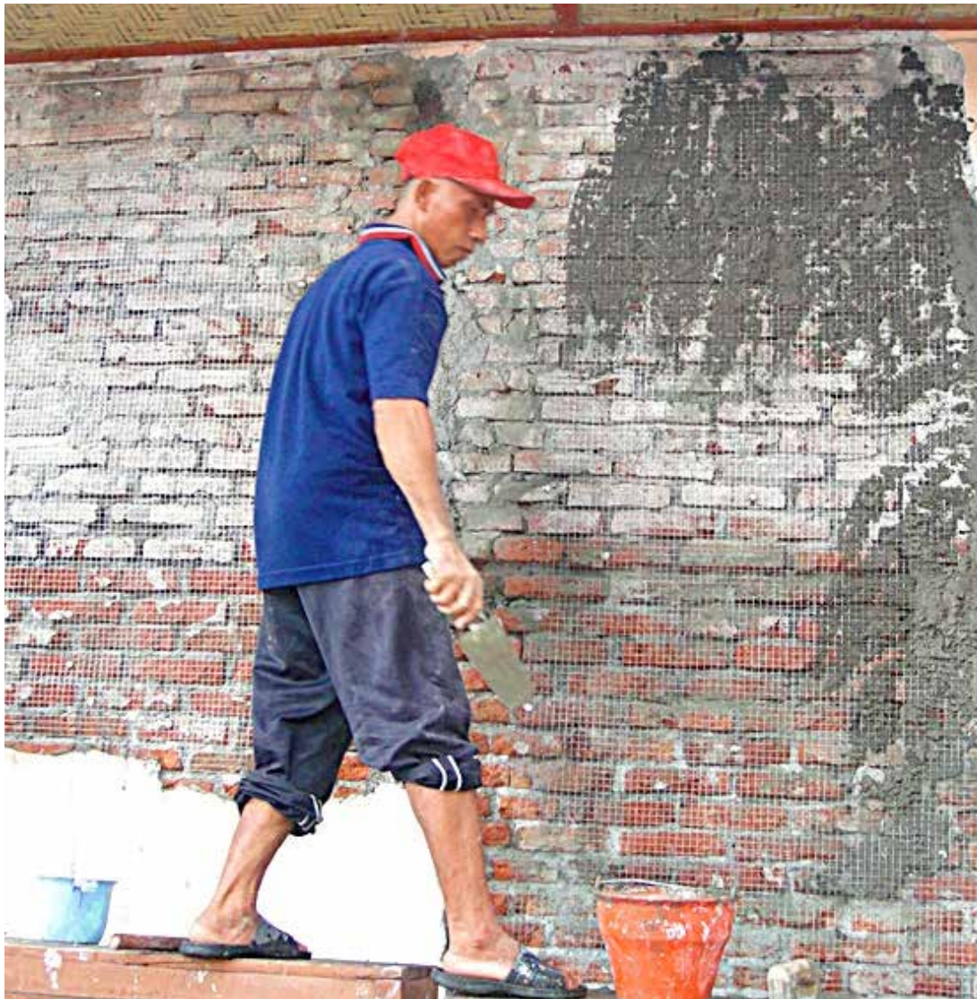
Wall reinforcement with wire mesh by retrofitting metode
