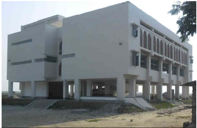
Completed School-cum-Cyclone Shelter, Bangladesh.
