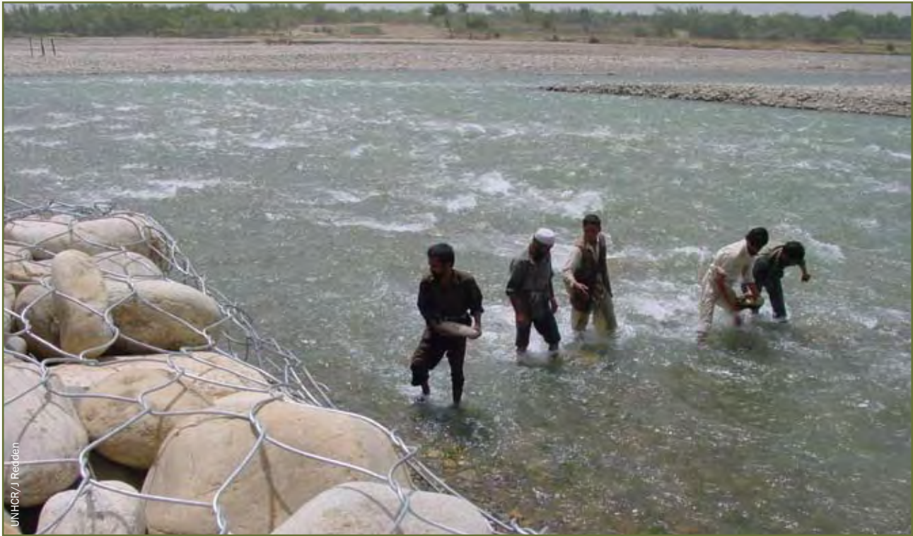
Returnee refugees building flood protection for Kalota, Kapisa Province, along Panjshir River, Afghanistan.
