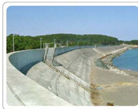
Sea wall with stairway evacuation route used to protect a coastal town against tsunami inundation in Japan. Photo courtesy of River Bureau, Ministry of Land, Infrastructure and Transport, Japan.
